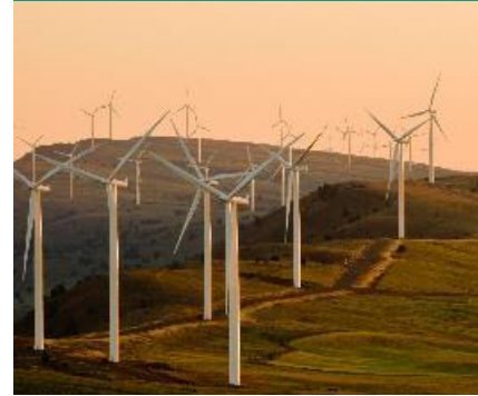
Process, Energy & Water
