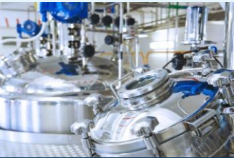
Equipment and products for pharma production
